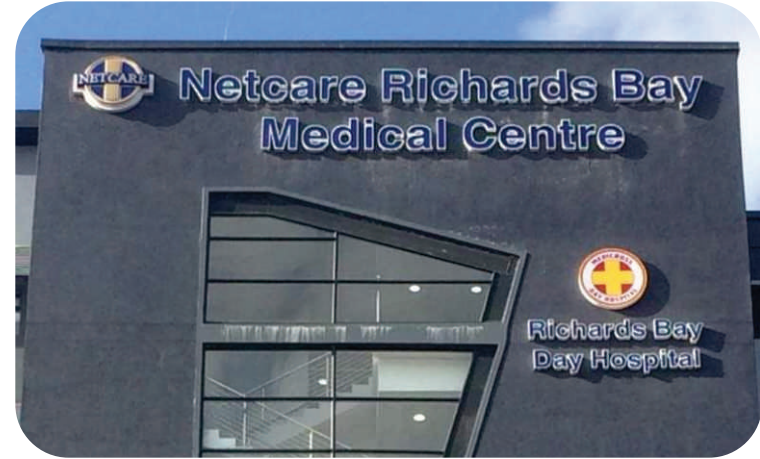
Fabricated 3D letters Perspex return, Perspex face, Led illumination.
