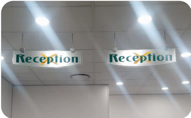
Profile cut glass with sandblast vinyl and colour vinyl decal. Hanging clamps.
